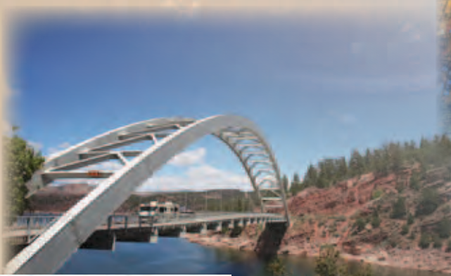
Cart Creek Bridge
